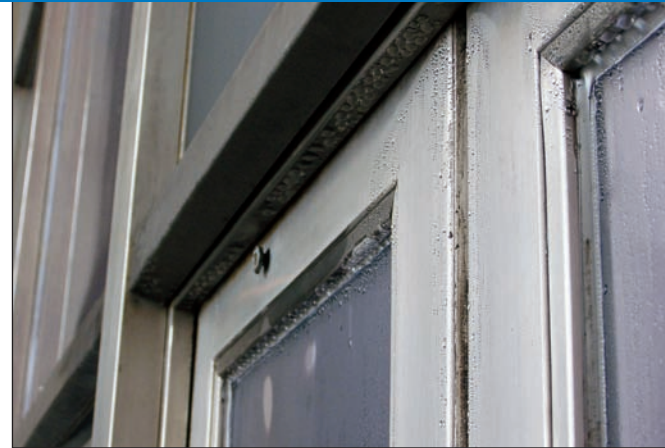
The photo above shows cold doors in insulated curtain walls, along with the resulting condensation on their interior surface.
