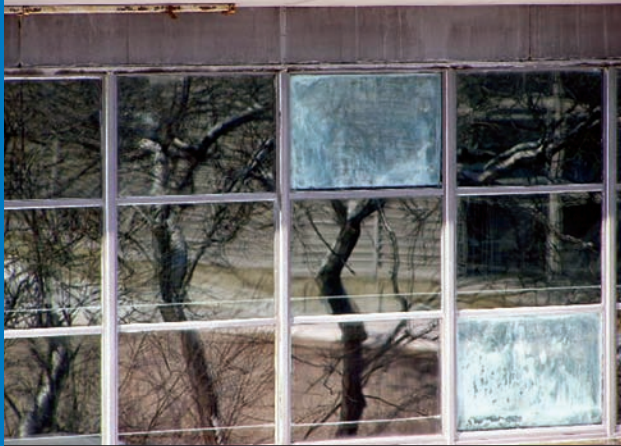
Airtightness is seldom achievable—the typical warranty on an insulated glazing unit (IGU) seal is 10 years.
